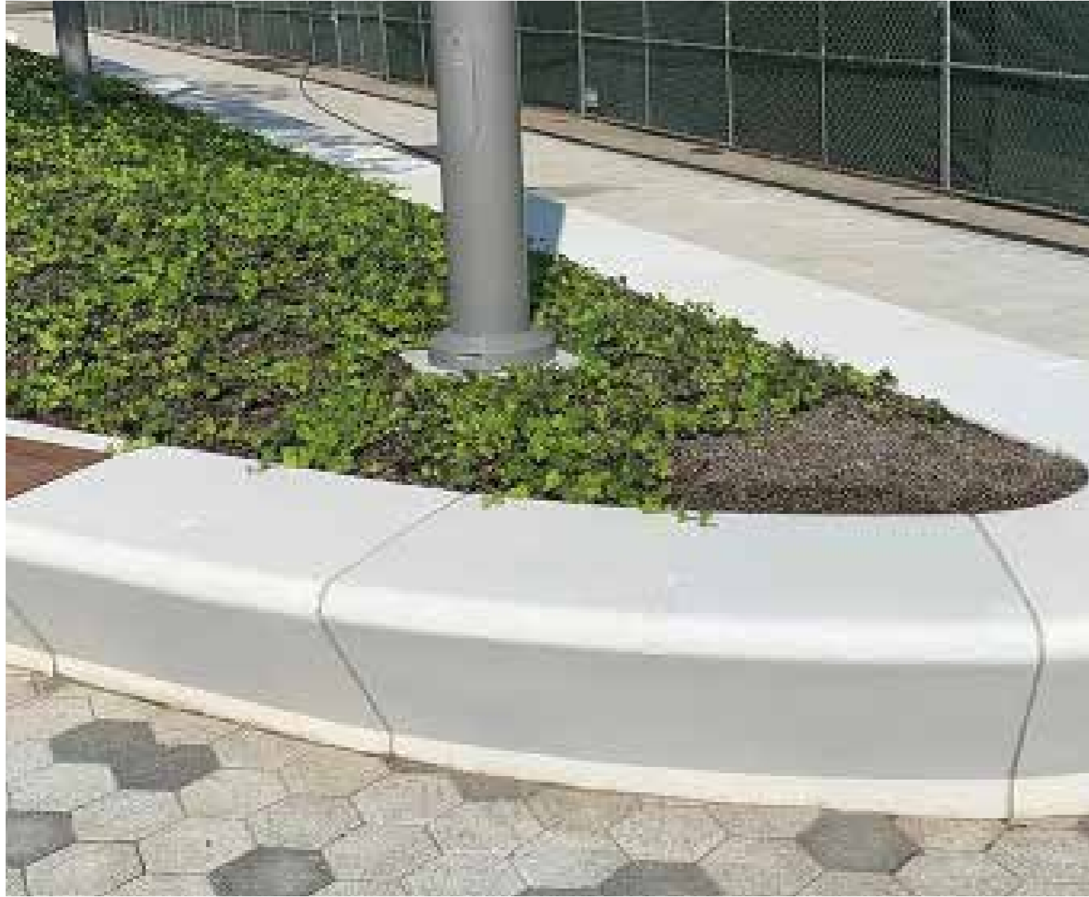
Curved concrete benches to form the entrance of the site
