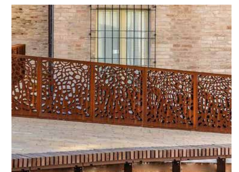
Laser cut corten steel panels can be used as fencing or inset into concrete
